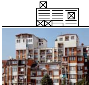
URBAN REGULATORY PLAN dating from 1978 - Number of full storeys 8-12 in fact 15 storeys - Uncontrolled stability of the construction - Commercial occupancy of common spaces for the dwellers
